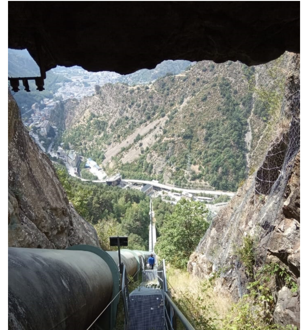
Maintenance of the penstock of the hydroelectric power plant.
