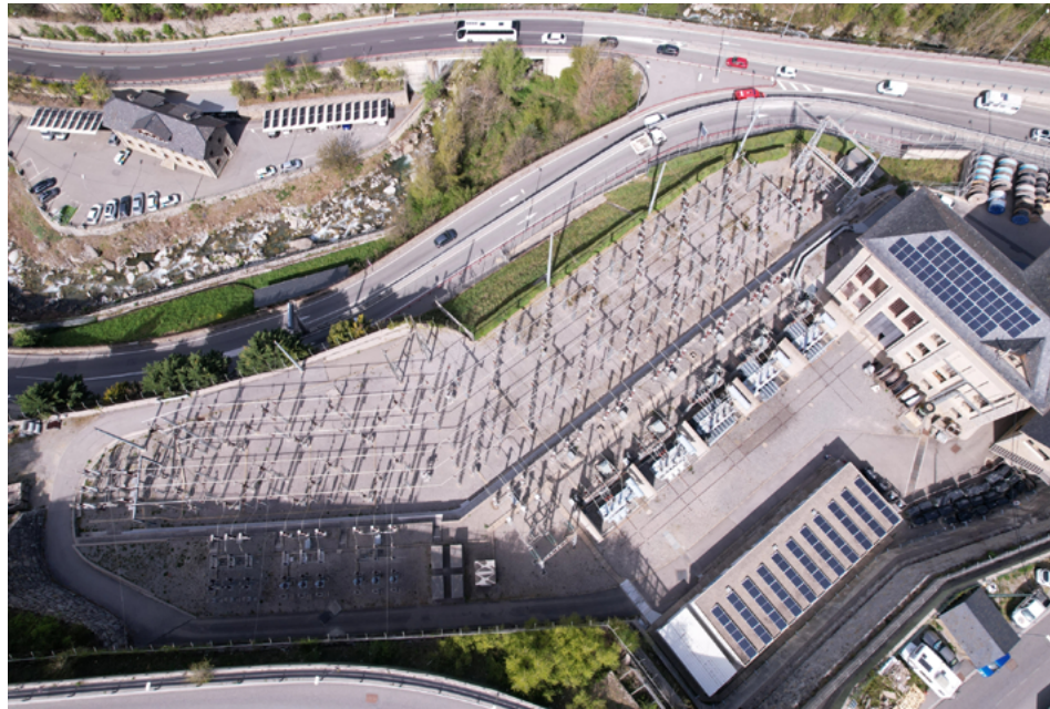
Photovoltaic installations at the Encamp ETR.
