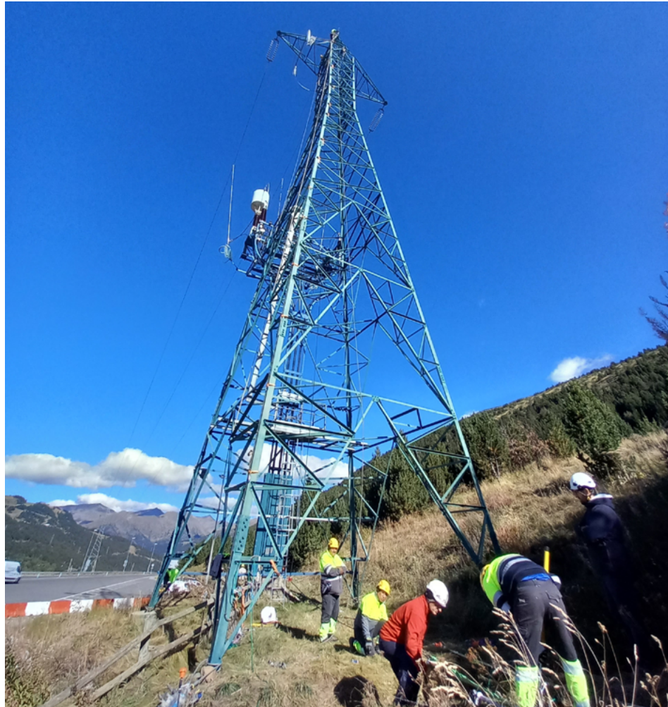
Dismantling of the old Encamp - Grau Roig high-voltage line.
